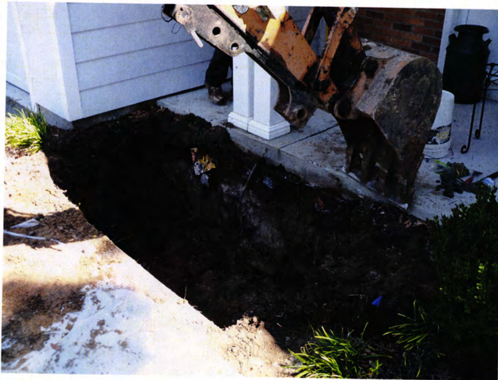
Picture 2: UST 141LaurelBB excavation in progress.
